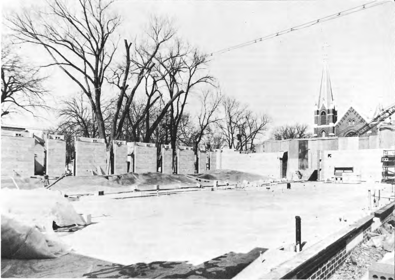
March 15, 1964 — Footings Completed
