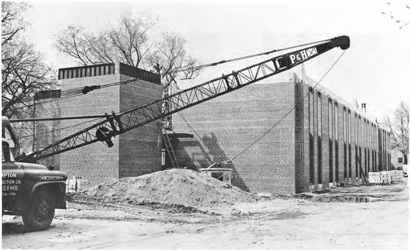
May 5, 1964 — Walls Completed
